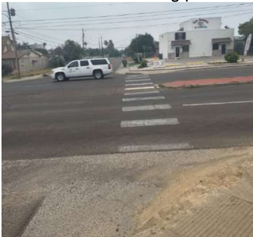
Figure 18: Difficult crossing across Clark Blvd with misaligned curb ramp
